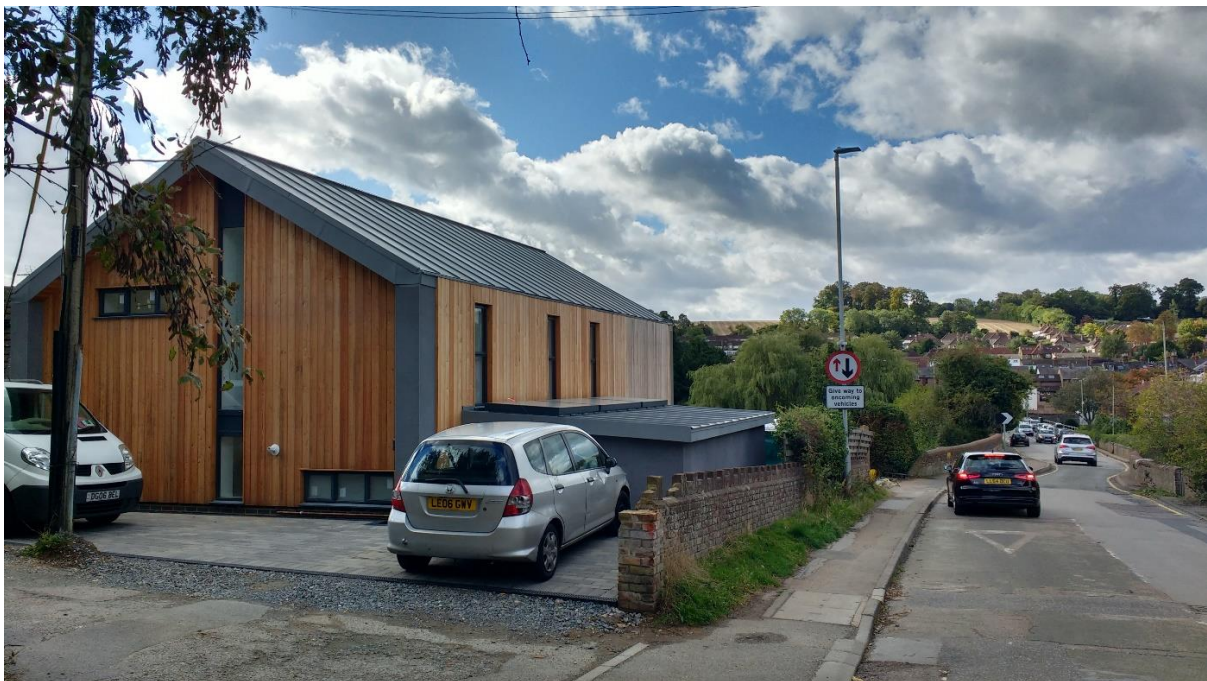
No.1 South Bank Road (ref: 4/02261/15/FUL) is located at a comparable gateway site
